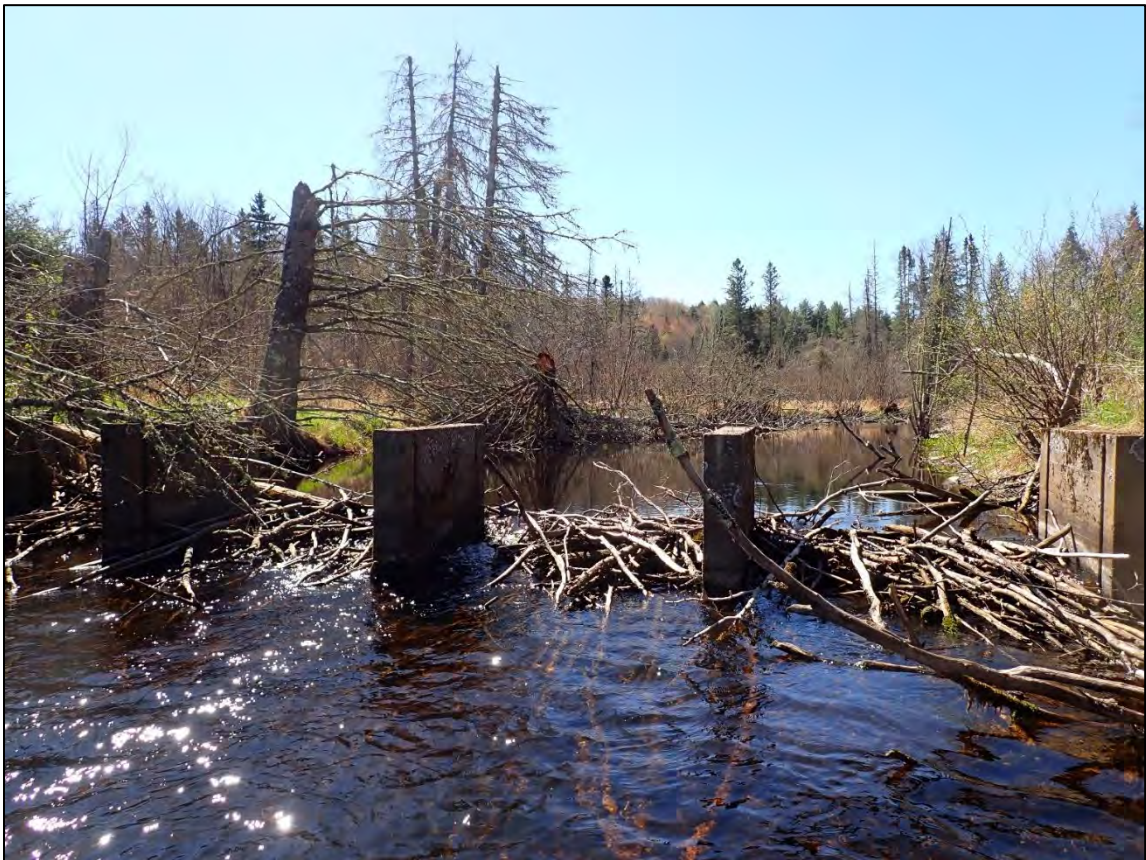
Photo 4. Concrete abutments of a remnant dam.
